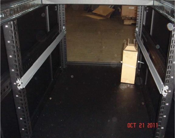
Make sure the rack rails they all secured in placed.
